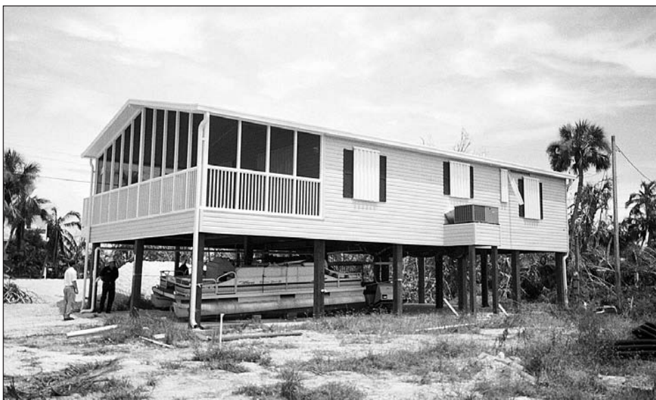
Figure 8-4. Manufactured home on a pile foundation.
